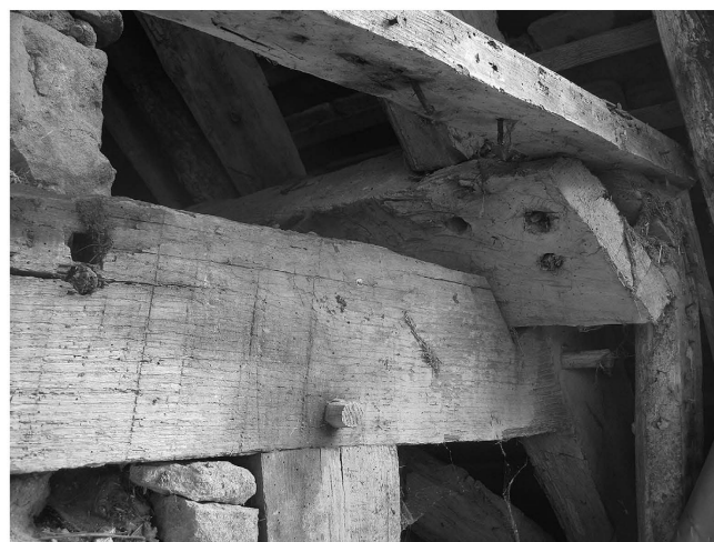
Fig 4. Detail of framing at south gable.
